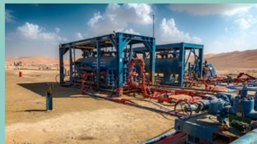
Zero flaring well testing: cutting methane, creating value
