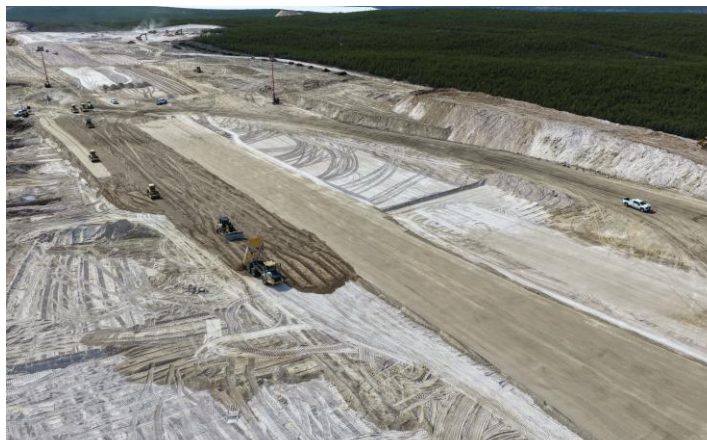
Airstrip Fill Placement
