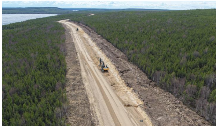
On-site Access Road
