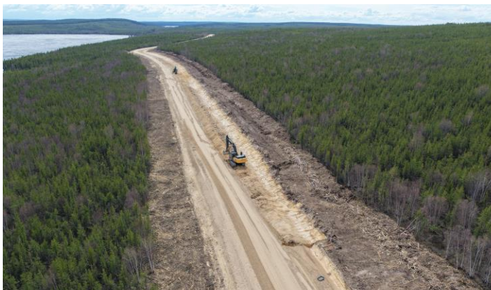
On-site Access Road
