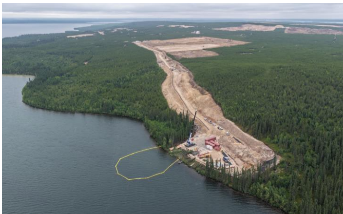
Diffuser Installation and Access Road
