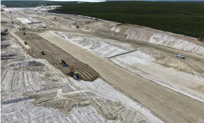
Airstrip Fill Placement
