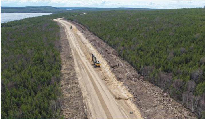
On-site Access Road
