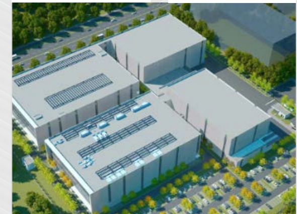
New Aptar Suzhou Facility
