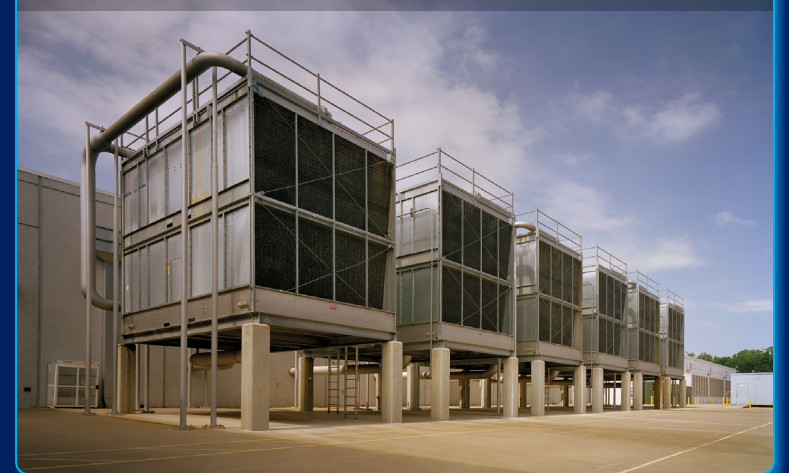
Concurrently Maintainable Chillers, Pumps and Cooling Towers
