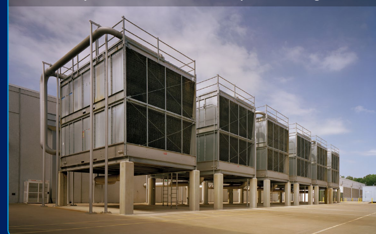
Concurrently Maintainable Chillers, Pumps and Cooling Towers
