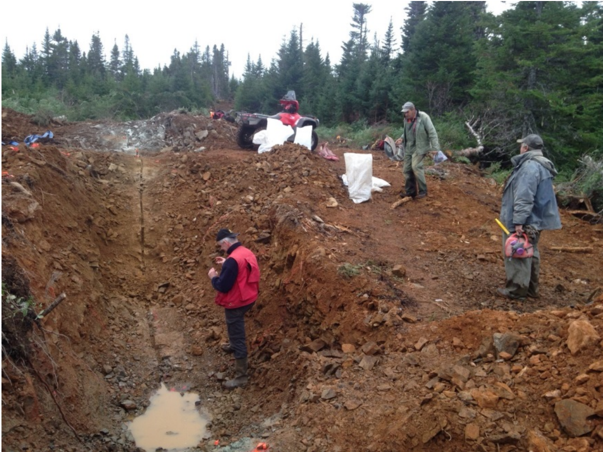
Plate 9: Highly Visible and Characteristic Intense Fe-Carbonate Alteration Associated with Gold Mineralization, Argyle Zone.
