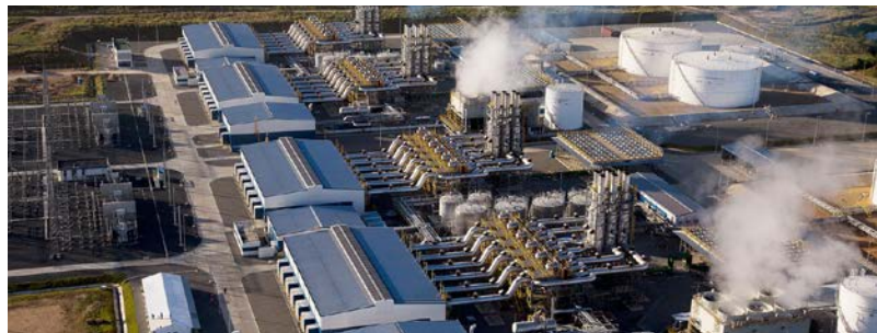
Above: Quisqueya power plant, Dominican Republic
