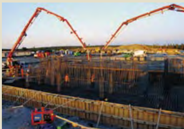
Sag mill foundation preparation at Canadian Malartic site
