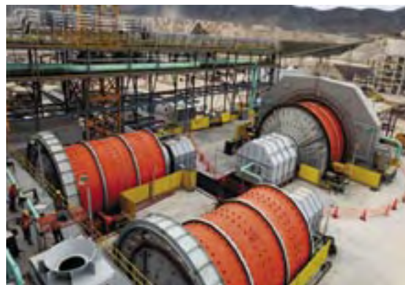
Construction of the Peñasquito grinding circuit
