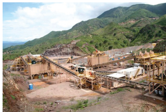
The crushing facility at the Dolores Project
