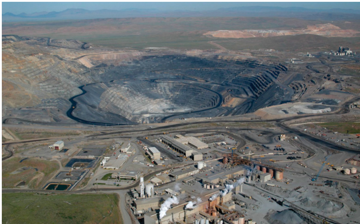
Aerial view of the Goldstrike mine
