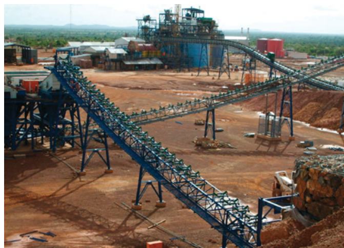
A view of operations at the Taparko mill
