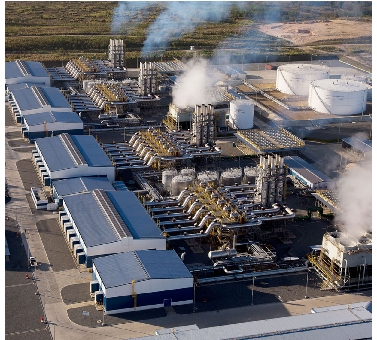
Quisqueya power plant, Dominican Republic
