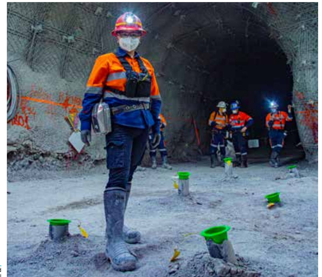
Drill hole preparation, underground undercut apex level
