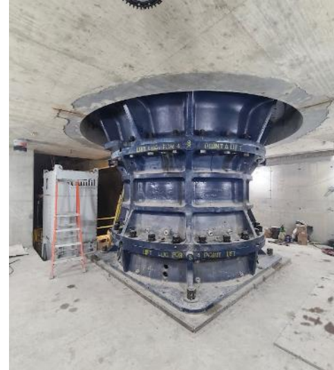
Mid shell of Gyratory Crusher
