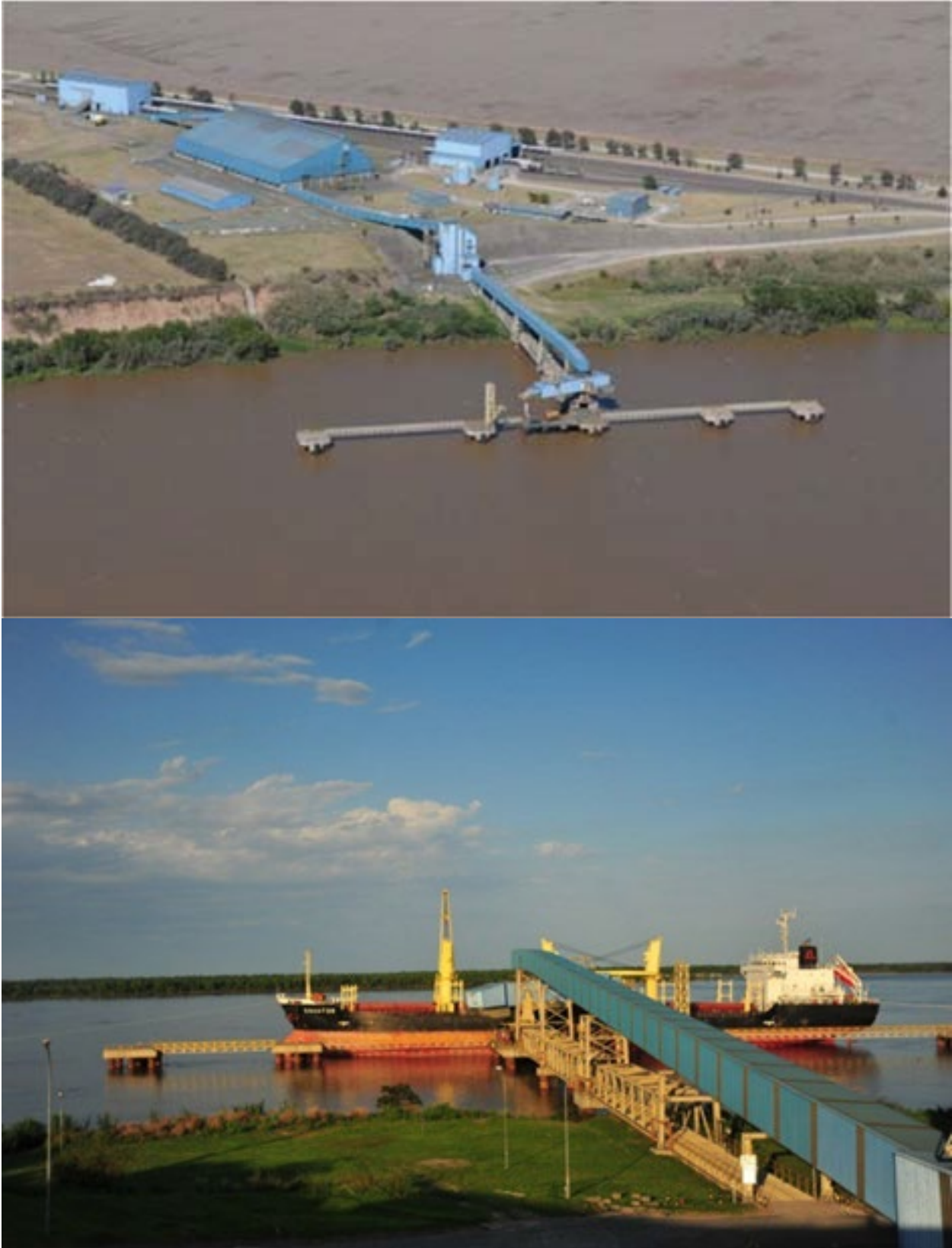
Figure 18-4: Ship Loading Facility
