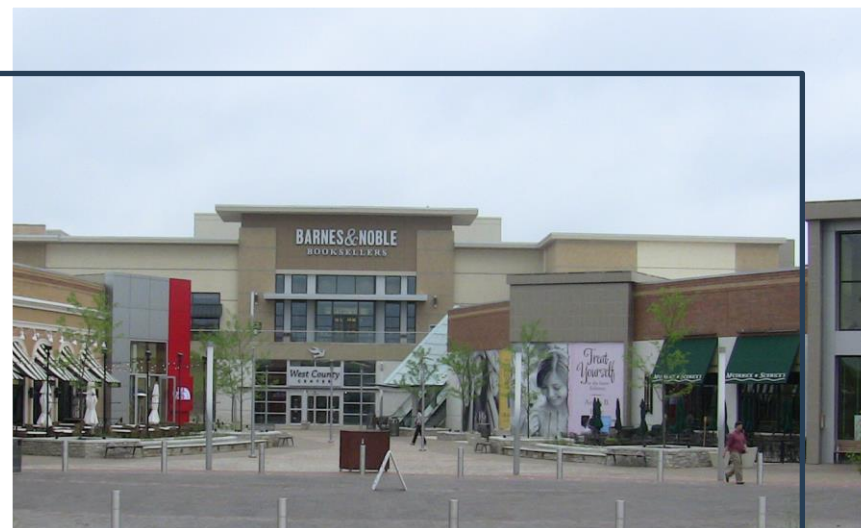
West County Center, St. Louis, MO
